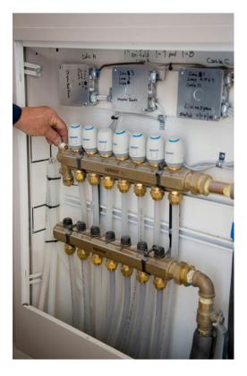
According to the National Association of Home Builders (NAHB) Research Center Design Guide, PEX pipe is efficient to install because it is flexible and uses mechanical fittings, eliminating the need for soldering and the flames and chemicals associated with "sweating" joints. It also resists corrosion and scaling. A PEX plumbing system is also cost effective because it is less labor intensive and can optimize system performance.
